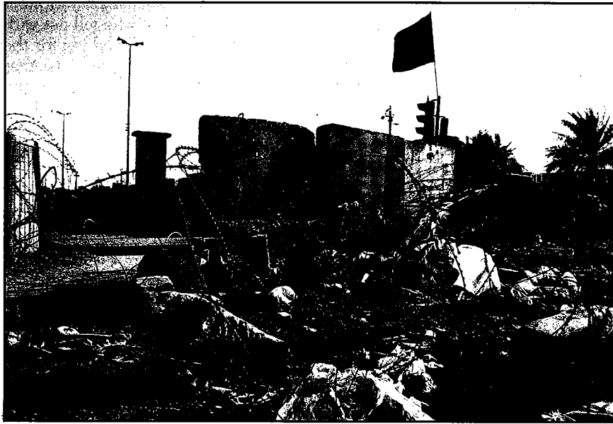
A BLAST WALL TO PROTECT AGAINST EXPLOSIONS
